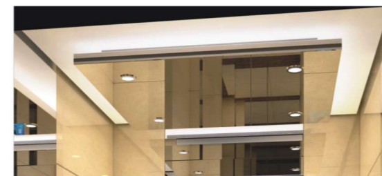
Lighting: mirror stainless steel ceiling panels, surrounded floodlights and direct flush lighting.
