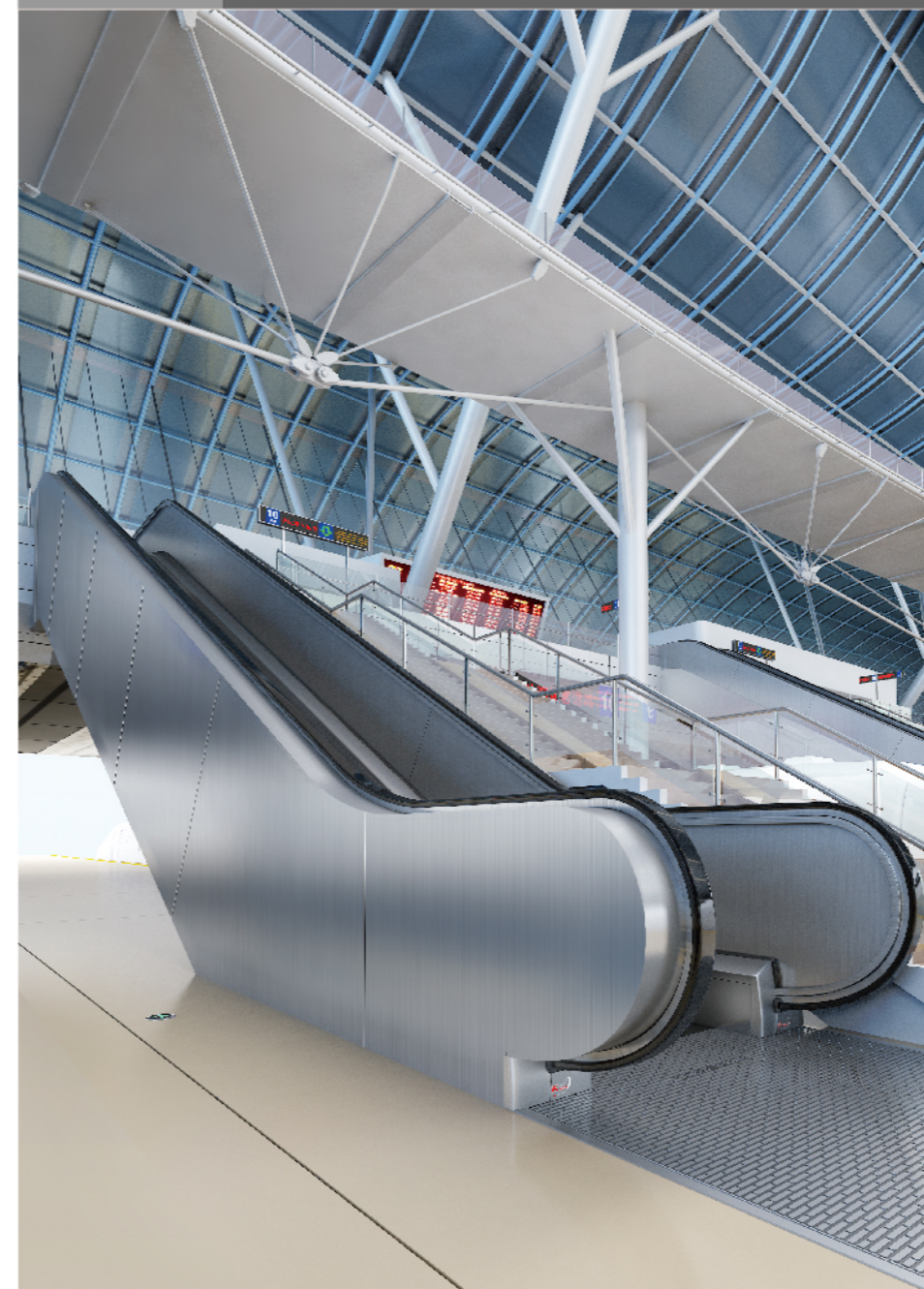
Plan 3-1 Stainless steel interior plate, external decoration plate perpendicular to step operation direction without lighting.
